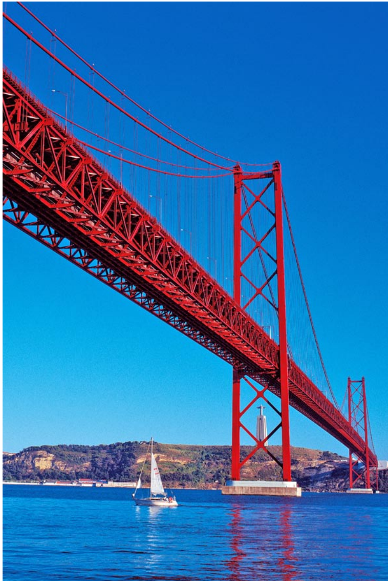
At the Tejo Bridge in Lisbon, a suspension bridge with extraordinarily high accumulated displacements, in autumn 2004 the damaged roller bearings were replaced by MSM® Spherical Bearings.
