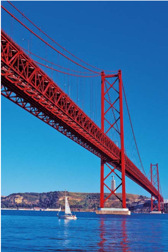
The bridge „Ponte 25 de Abril“ links Lisbon with Almada. At the 2 abutments and at the cable bearer piers, roller bearings were replaced by MSM spherical bearings
