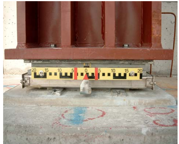
Fig. 3, 4: supporting point of cantilevering steel truss beams, MAURER MSM ® spherical bearing
