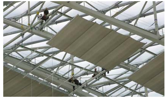
Fig. 1-3: installation of protection curtain system
