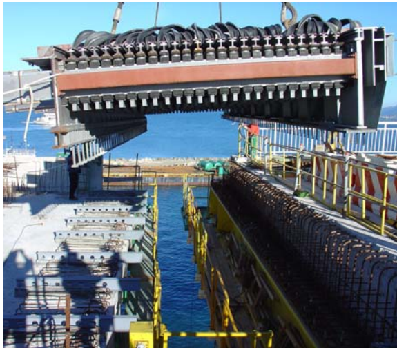
Fig. 1, 2: Installation of the Rion-Antirion expansion joint
